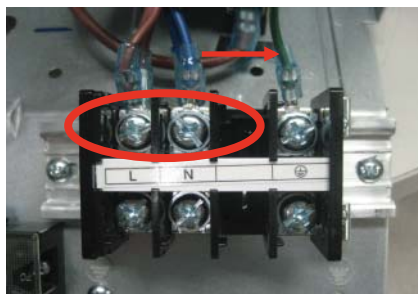
< Input Power Source Check Point >
