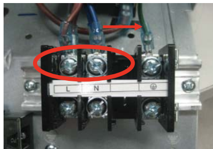
< Input Power Source Check Point >
