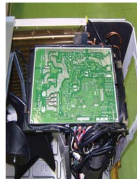
Tighten PCB Screws (4ea)
